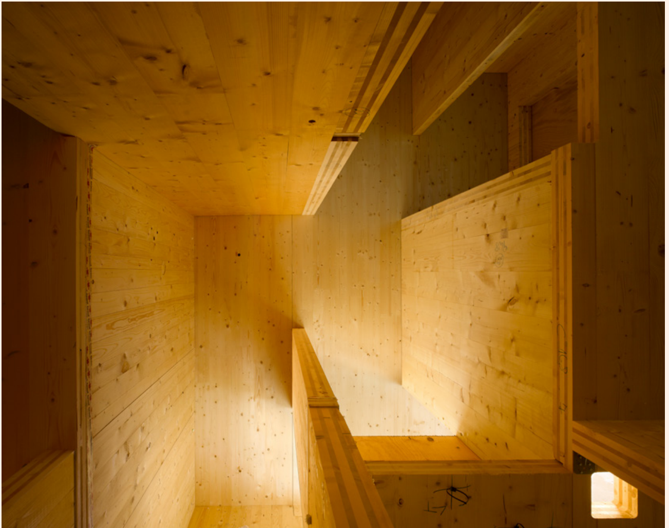
Murray Grove – the first urban housing project to be constructed entirely from pre-fabricated solid timber. Image: © Will Pryce
