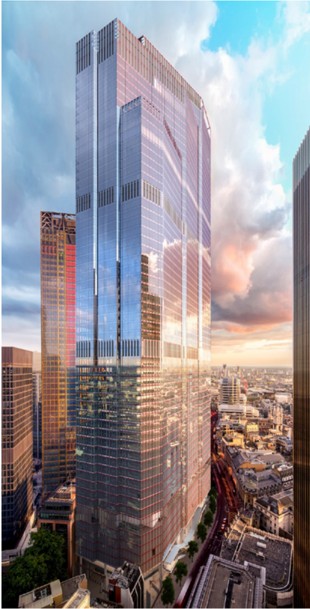
The construction of 22 Bishopsgate will also see a consolidation centre employed for the delivery of construction materials. Image: The Architects' Journal
